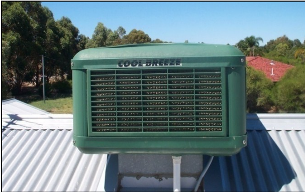
Figure 2. A roof mounted evaporative air conditioning unit. Figure 3. A cellulose filter pad exposed to ember attack (during testing)
