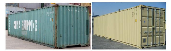
Above left image: An unpainted sea/shipping container that has visible rust, worn paint and has wear and tear damage/denting. Is only considered appropriate for approval where it is:
