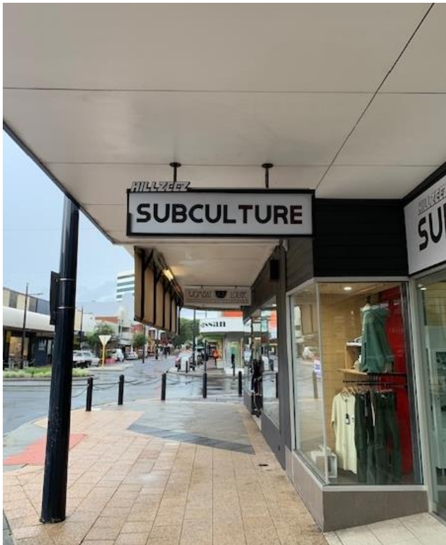
Above: A shop with an acceptable under verandah sign.
