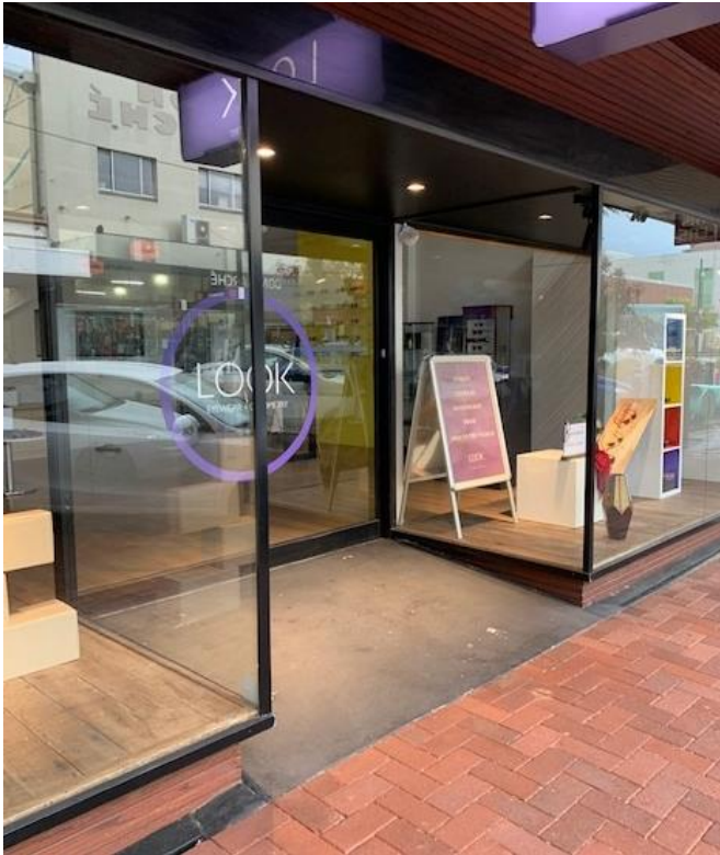
Above: A shop frontage with a recessed entry point and adequate glazing.
