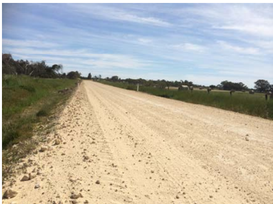
Trotter Road Re-sheeting
