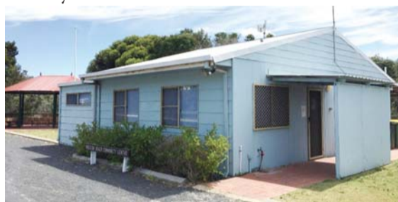
The existing Community Centre on Panorama Drive in Preston Beach
