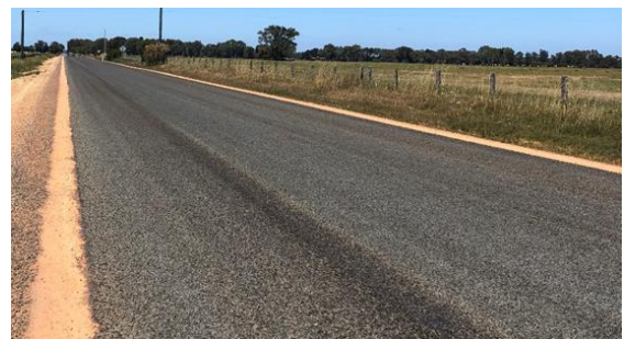
Photo 20: Somers Road reconstruction
