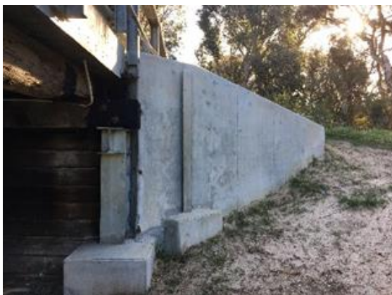
Photo 22: Repairs to Lake Clifton Road bridge
