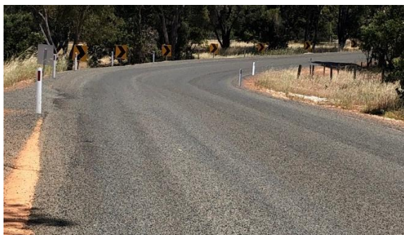
Photo 21: Southern Estuary Road reconstruction
