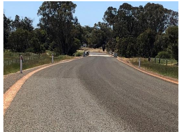
Photo 19: Coronation Road reconstruction
