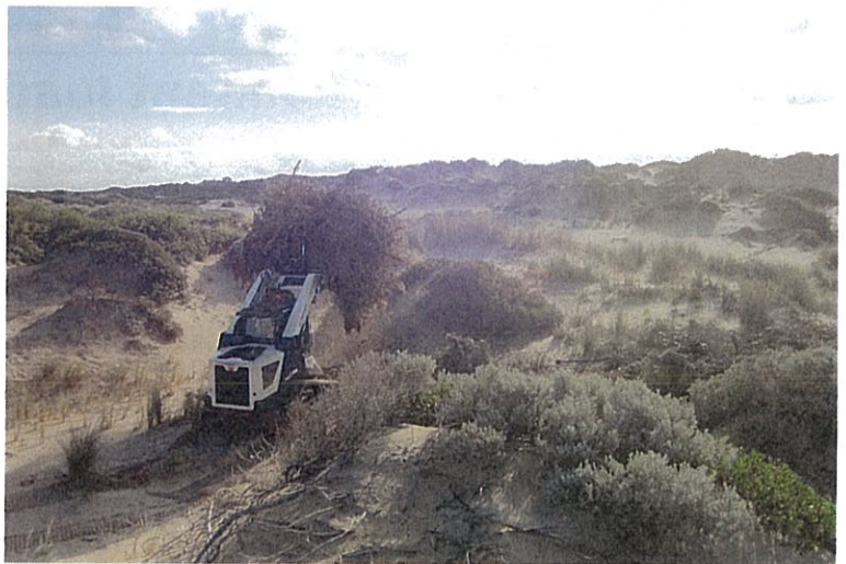
• Positrack machine laying dune brushing
